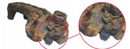
Starke Korrosion / strong corrosion
